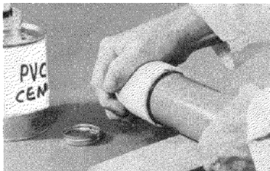
FIG. X3.4 Assembly of Joint
